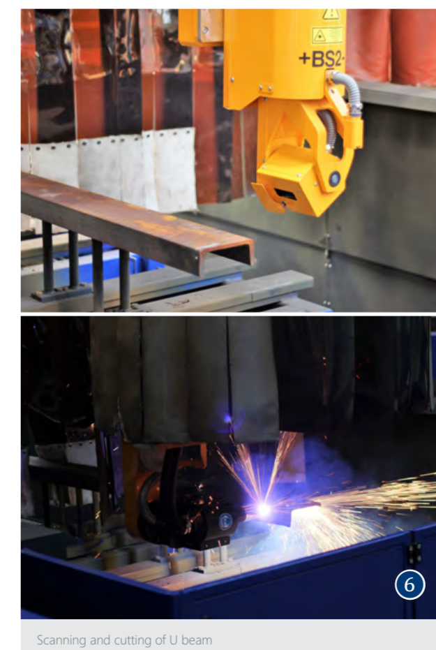
6 Scanning and cutting of U beam
